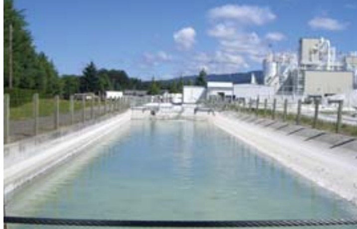
CRC's new wastewater treatment facility handles all process wastewater and recycling, storage, loading and transport of agriculture lime by-product.
